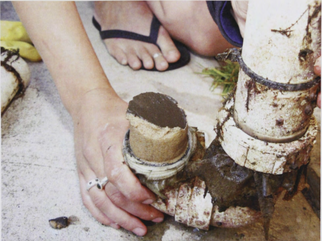
Figure 5.6: Sand filter over meshing in PVC pipe, trapping fine grained material in the seawater.
